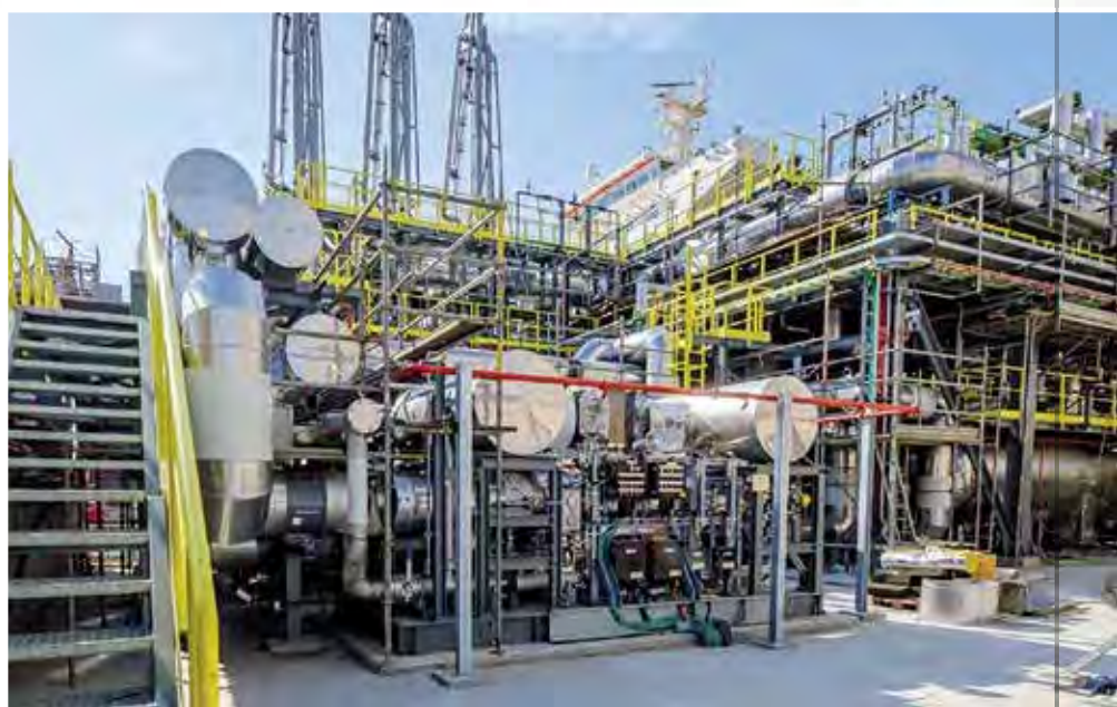
BOG compressors - Courtesy of DIG (Depositi Italiani GNL - Italian Coastal LNG Deposits), Ravenna, Italy
